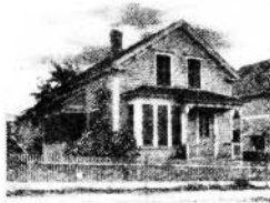
A No. 3-22 IDEAL Boiler and 400 ft. of 34-in. AMERICAN Radiators, costing the owner $195, were used to Hot-Water heat this cottage.
